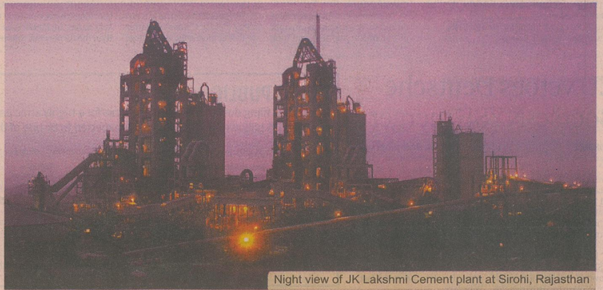
Night view of JK Lakshmi Cement plant at Sirohi, Rajasthan
